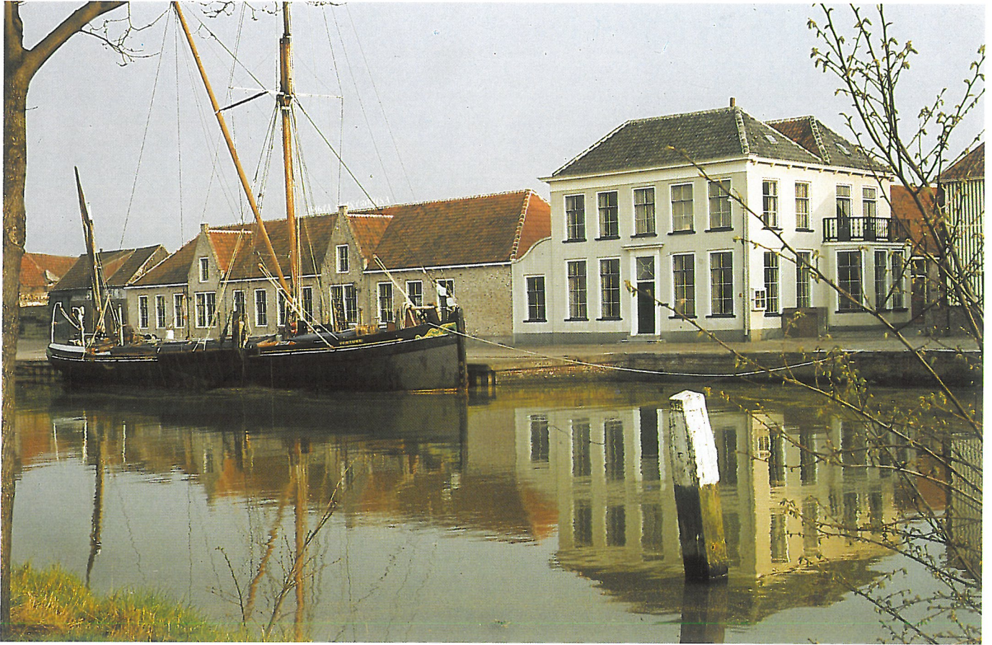
The restored historical buildings where Delta Elektronika B.V. have their offices, development department and part of the production departments.
